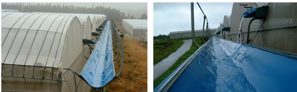
Fig. 4. The photos of running water on the rainwater collecting gutters at the Foundation Seed Production Center in Aewol-eup.
