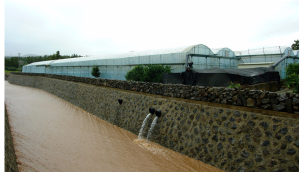
Fig. 6. The photo of discharging rainwater overflow from storage tank to stream at Hoecheon-dong.
