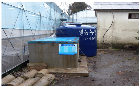
Fig. 8. The photos of rainwater harvesting facility composed of storage tank and artificial recharging system (left) and artificial recharge process (right).
